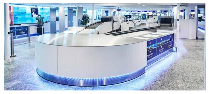
First, the four lanes feature a total of 10 parallel divest stations, enabling multiple people to prepare simultaneously for baggage screening. Second there is an automatic tray return, rather than traditional manual transfer back to the start; and thirdly automatic diversion efficiently separates suspicious baggage from the main conveyor.
